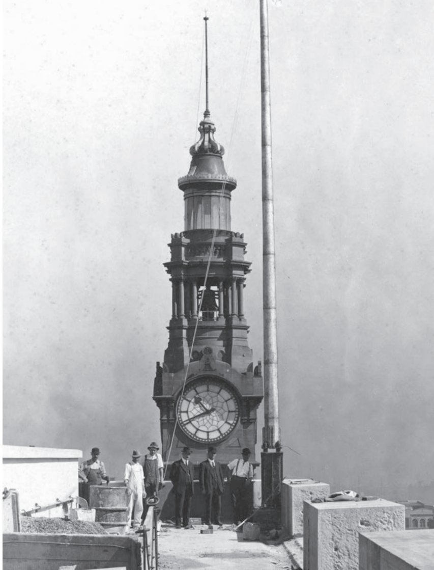
Erection of the flagpole on the roof of the Commonwealth Bank of Australia's head office, 12 April 1916, looking across to the clock tower of the General Post Office, Sydney.
