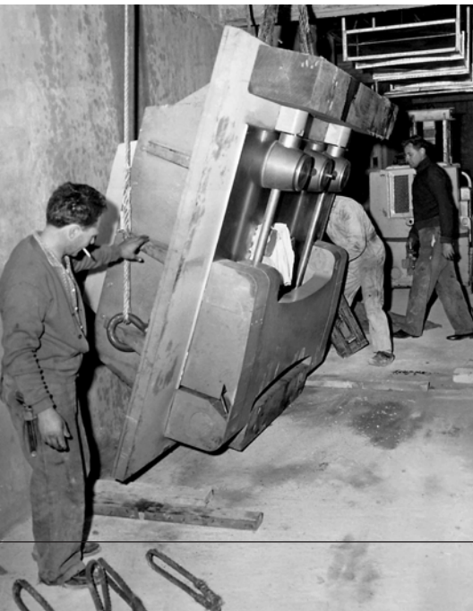
The doors of the strongrooms weighed 18 tons, and its walls were 75cm thick.
