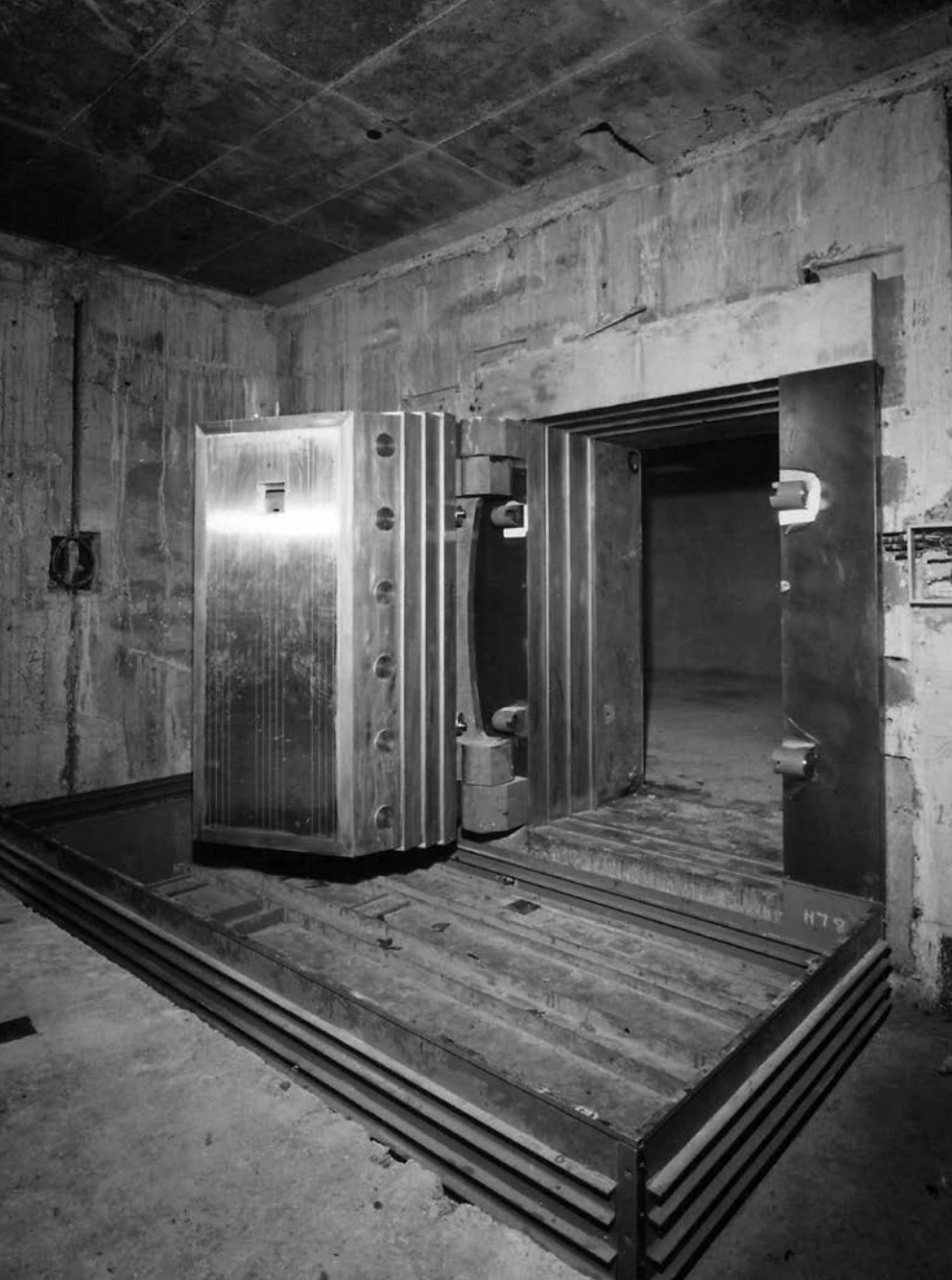
The installation of specially designed doors for the Bank's strong room; the door weighed 18 tons. Reserve Bank of Australia Archives. PN-011269, PN-011239.
